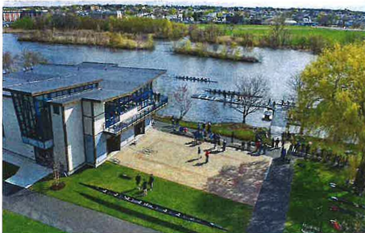
Tufts Boathouse with paved crew staging area and floating dock system.
