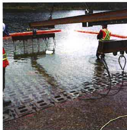
Example of the installation of articulated block mats at a boat launch.
