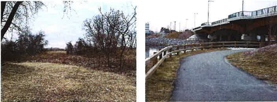
(Left) View to existing wetland looking north; (Right) New underpass trail at Route 16 bridge.
