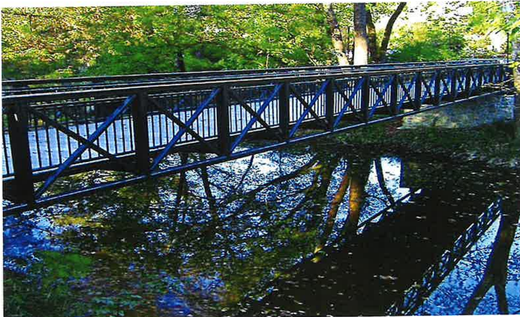
Example of prefabricated pedestrian bridge.
